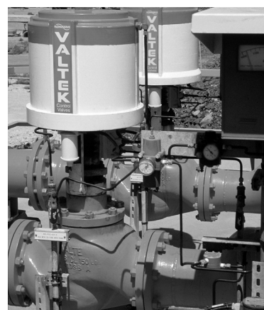
(right) A liquid nitrogen loading facility in Australia uses two Mark One valves for its emergency fire water system.
